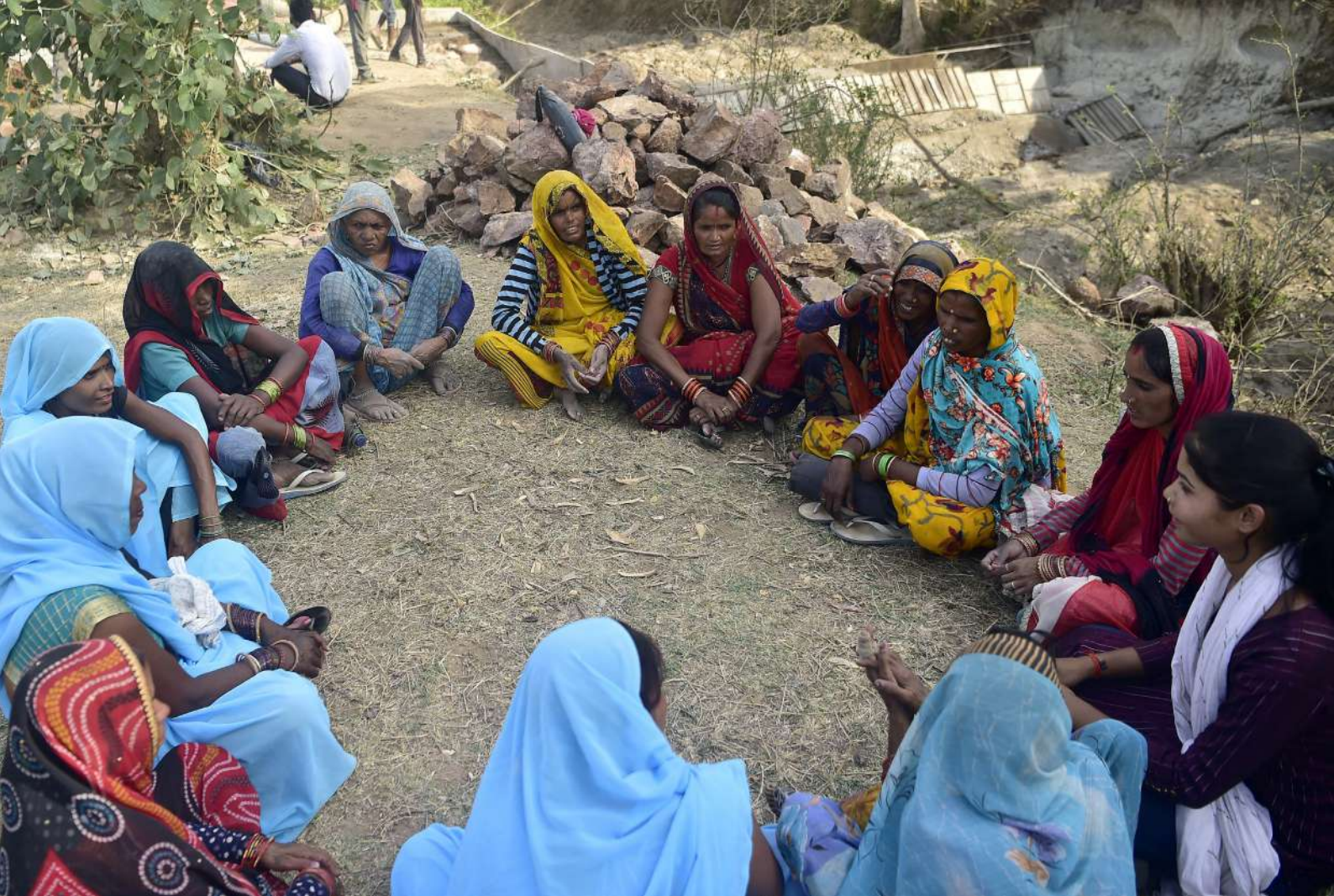
Volunteers from Jal Saheli Friends of water participate in the construction of a check dam on dried up Bachedi stream in Agrotha village, in Tikamgarh, Madhya Pradesh, India in June 2022 Photo credit: SANJAY KANOJIA/AFP via Getty Images
