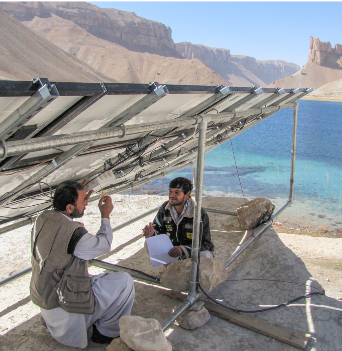
Technicians install and test a solar array as part of a project to electrify rural schools in Bamiyan province, Afghanistan. Credit: Robert Foster / Winrock International / US AID / CC BY-NC 2.0.
