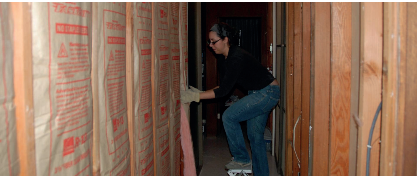
Installing insulation. Photo: Nick Nguyen
