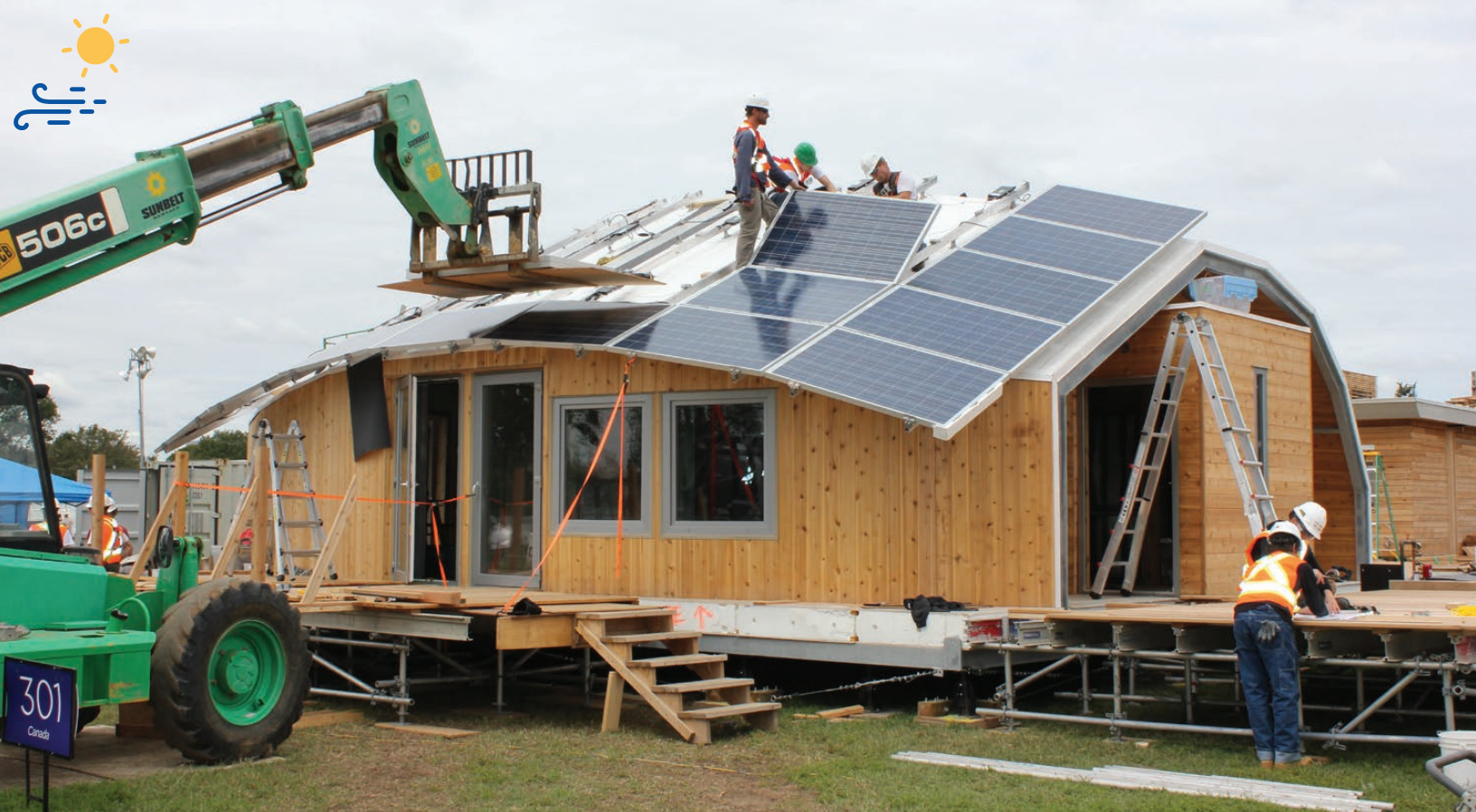
Installing solar panels on the roof of a Traditional Living house at the University of Calgary. Photo: Carol Anna/U.S. Department of Energy
