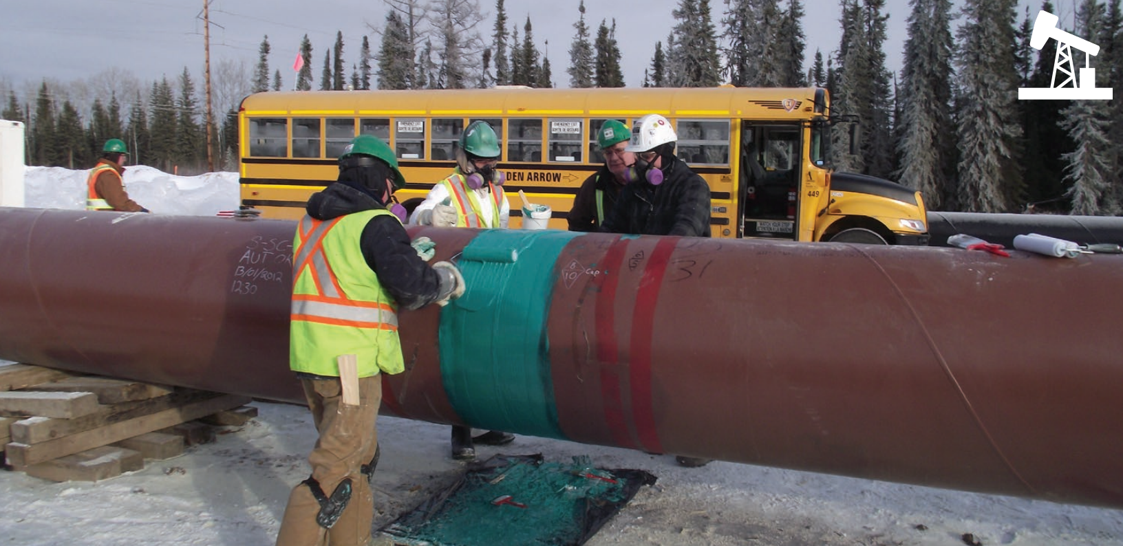
Albertan oil workers applying epoxy coating to a pipeline. Photo: jasonwoodhead23
